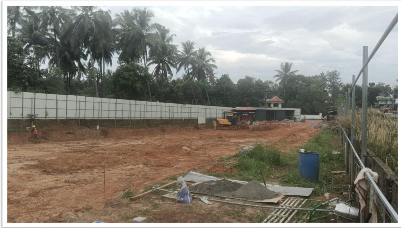
SITE WORK IN PROGRESS - VIEW 1
