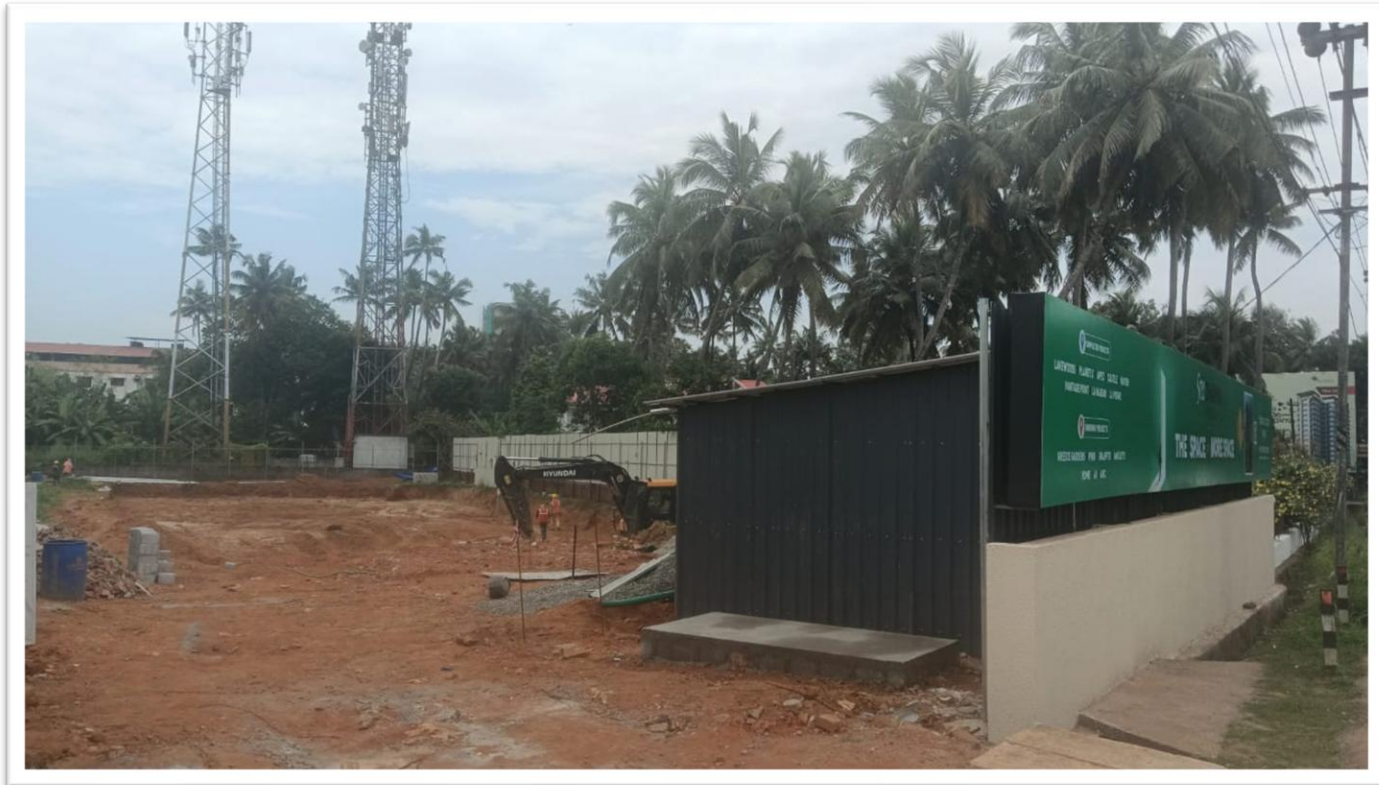
SITE WORK IN PROGRESS - VIEW 2
