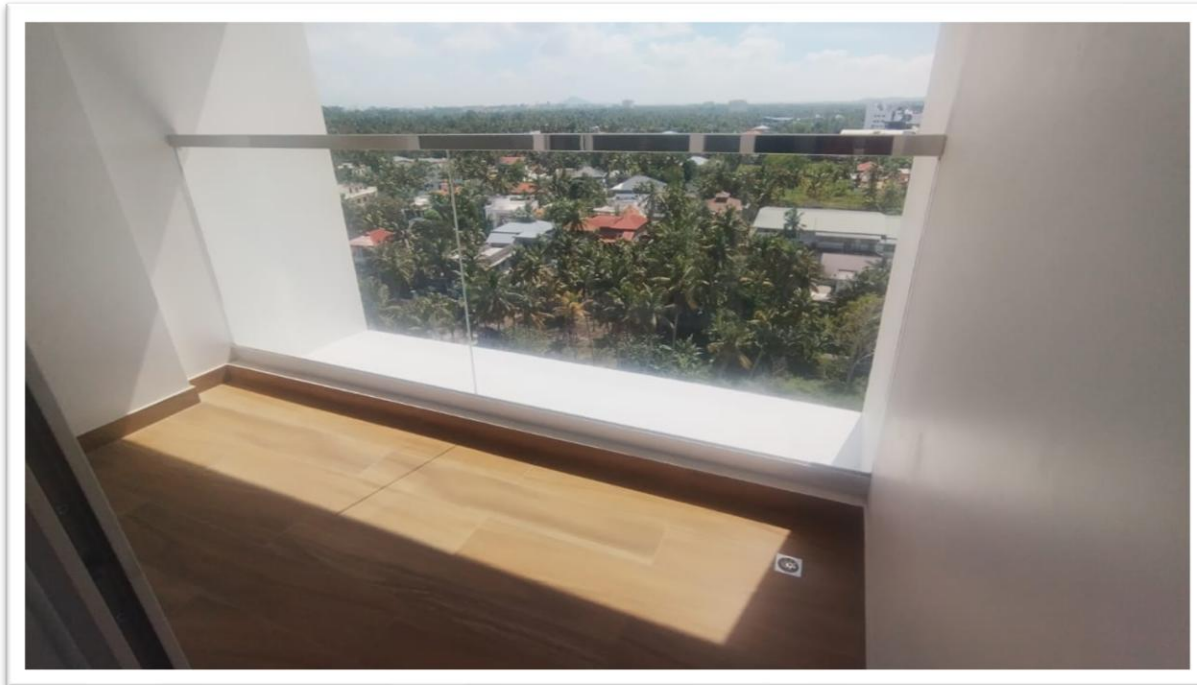
BALCONY FLOORING & HANDRAILS
