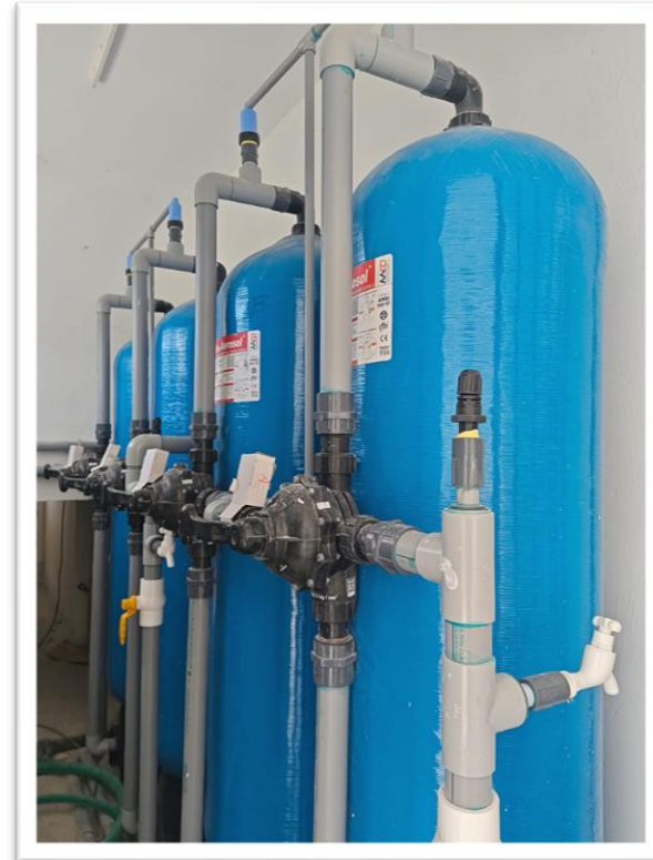
STP PUMP ROOM
