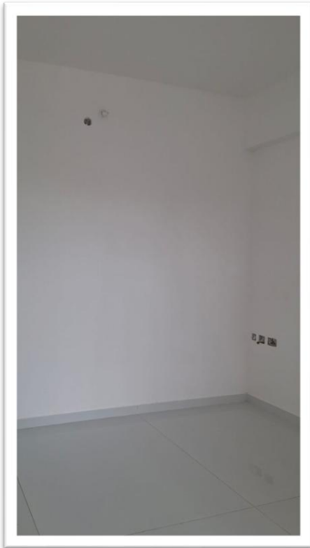
CEILING PLASTERING & PUTTY WORK
