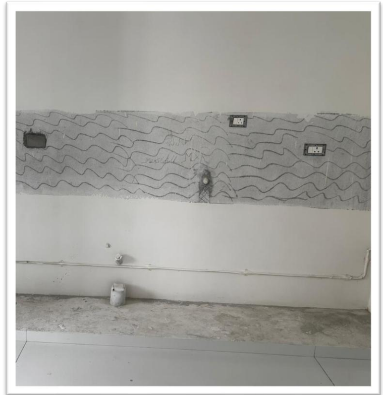
INTERNAL PLUMBING WORKS
