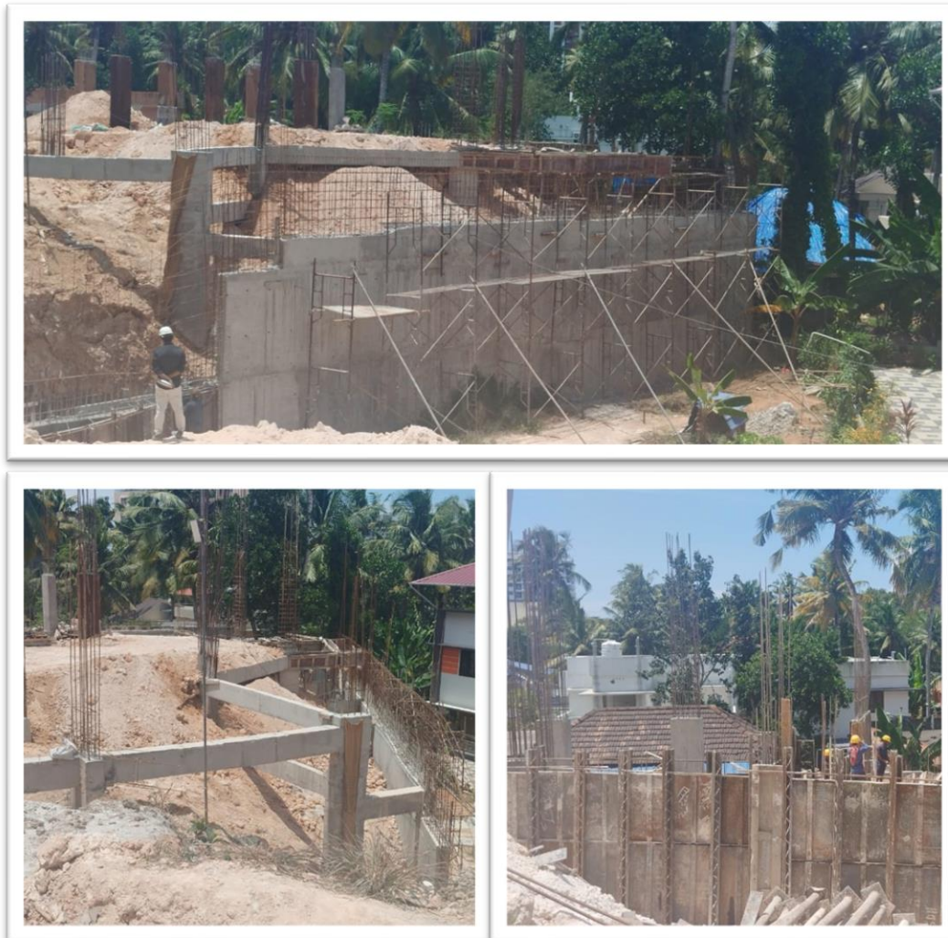
COLUMN FOOTING & RETAINING WALL
