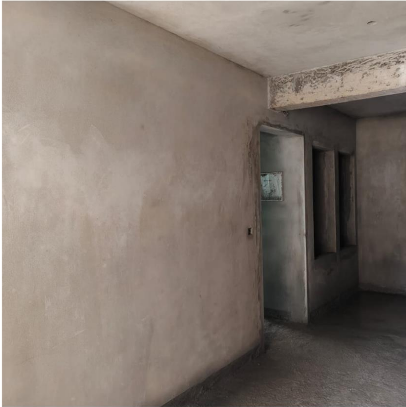
APT BLOCKWORK & PLASTERING
