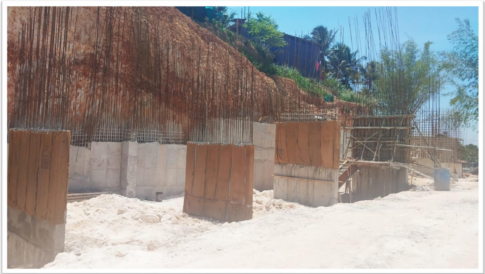
COLUMN FOOTING & RETAINING WALL
