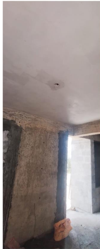
TERRACE CEILING PLASTERING & FLOOR
