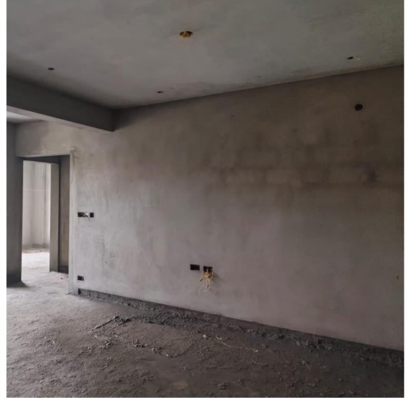
ELECTRICAL WALL CHASING & BOX FIXING
